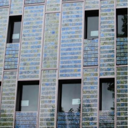
Figure 5.51: Integration of Photovoltaic Cells with Building Facade
