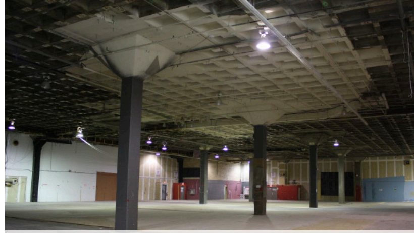
40 Carl Hall Road Interior building space
